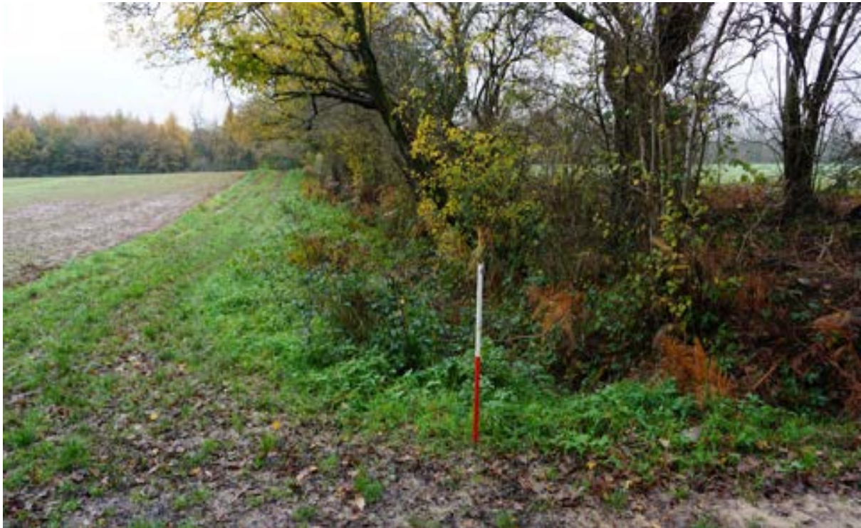
Plate 7.2: View southwards along historic field boundary to the south of Ansty Farm/The Place with bank and historic hedgerow ( B ) on west side (right) and flanking ditch on the east (left) – an historic trackway ( A ), now a farm track runs along the western side
