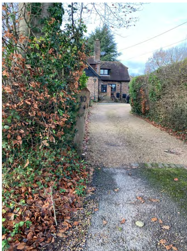
Figure 41: View down track of Wickham Barn
