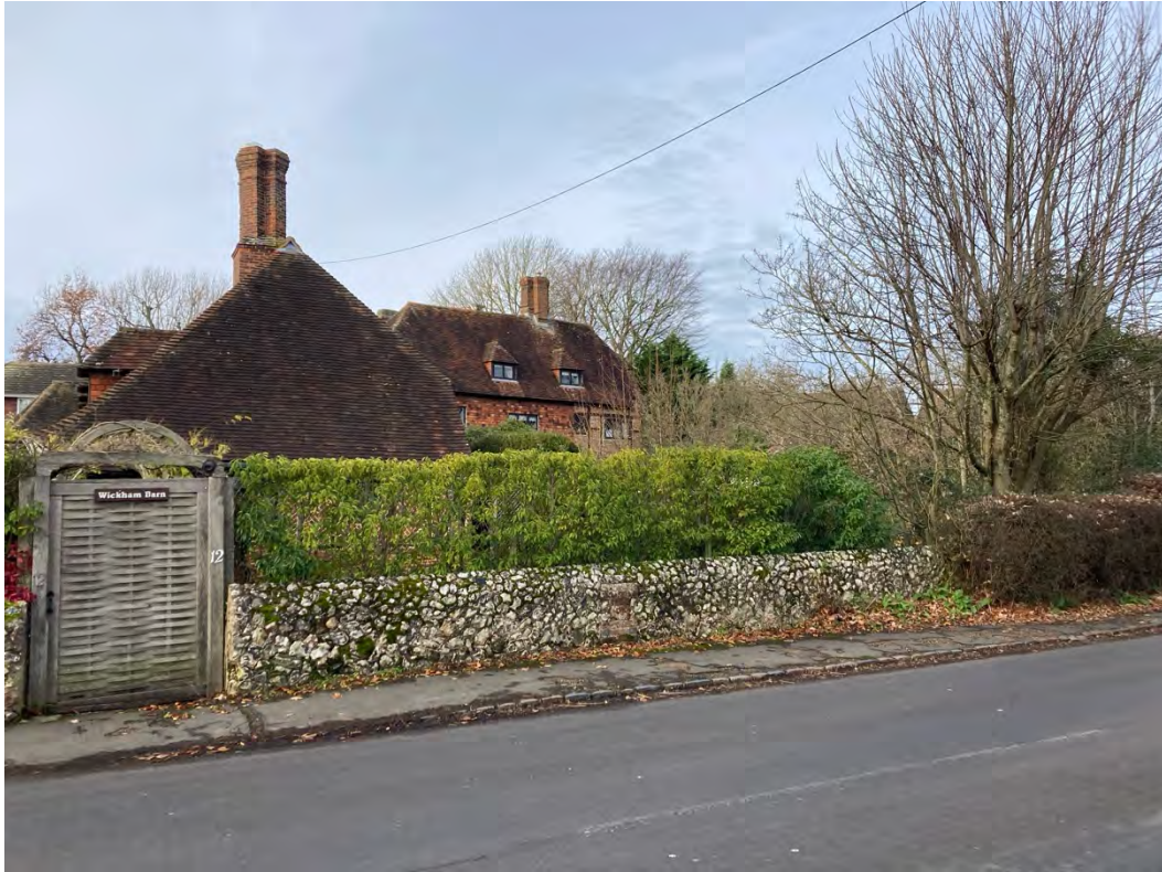
Figure 38: View from adjoining road of Wickham Farmhouse
