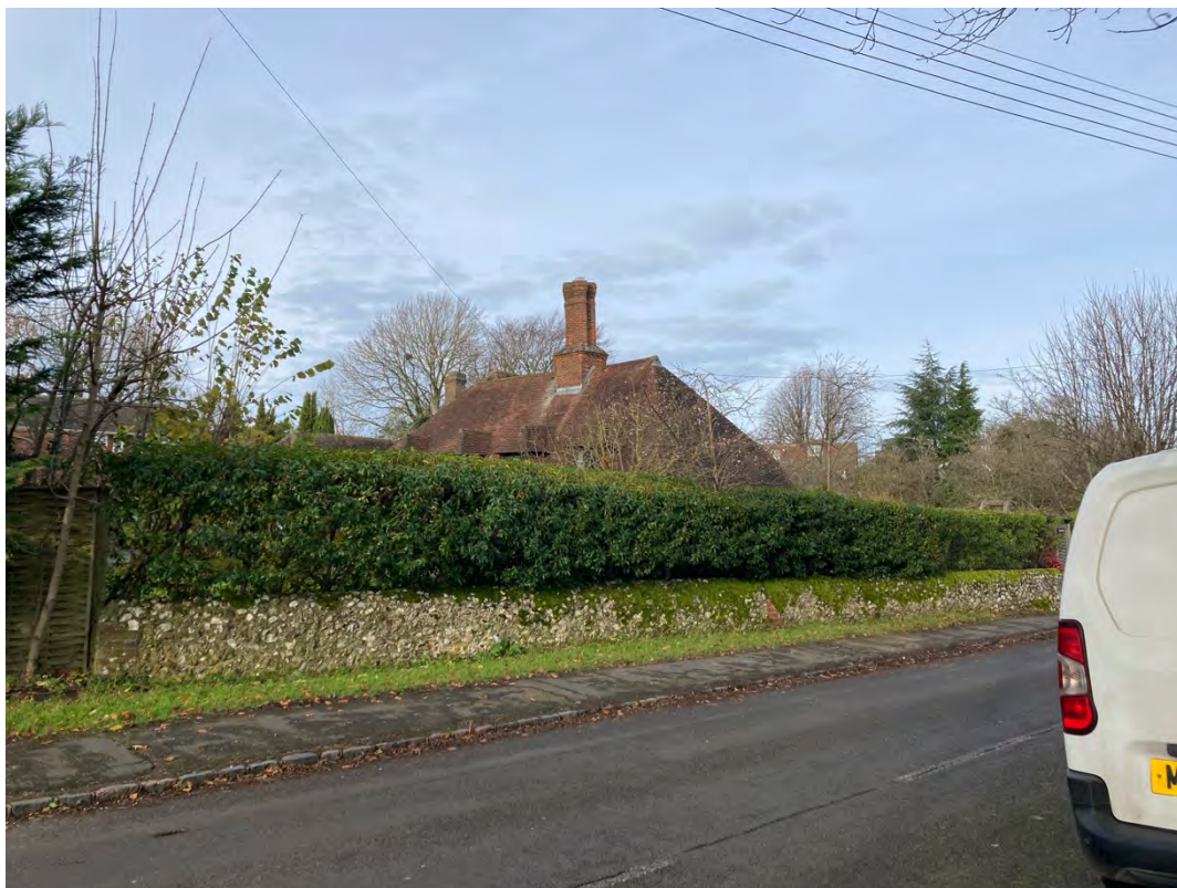
Figure 39: View from road of Wickham Farmhouse
