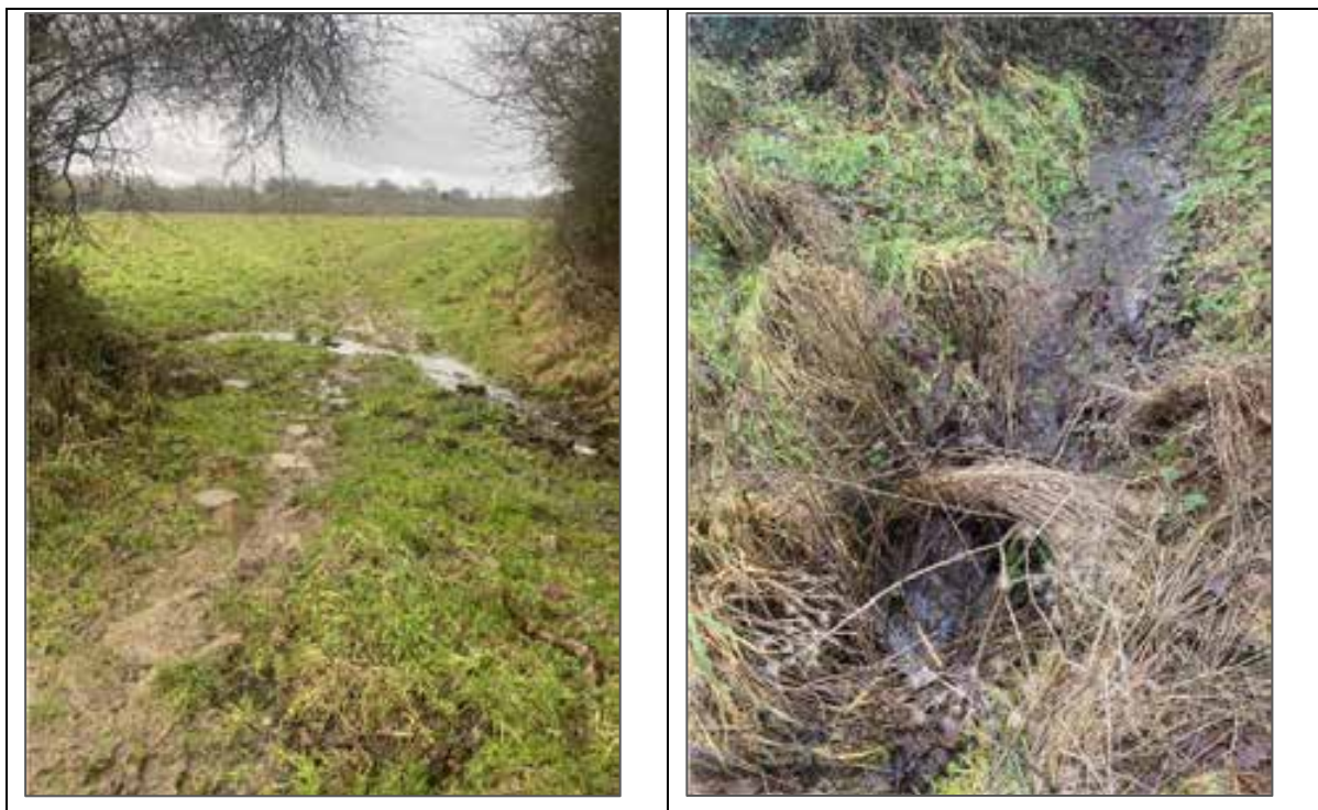
Figure 3-6 (Left) Drain 1 in the north (right) Drain 8
