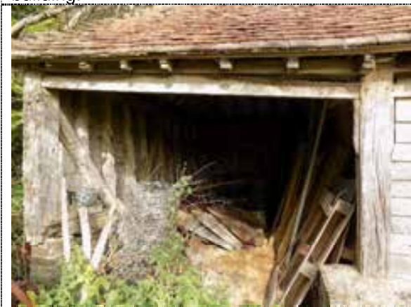
Figure 42: View of the western room
