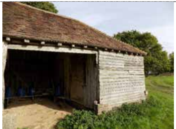
Figure 41: View of eastern room
