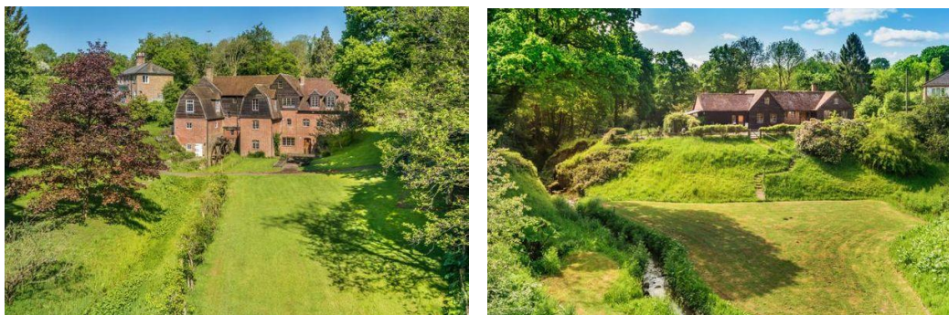
Figure 4.9: Highbridge Mill, south east (left) and north west (right) elevations 40
