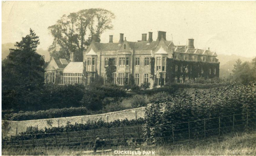
Figure 3.7: South elevations of Cuckfield Park, early 20 th century 19
