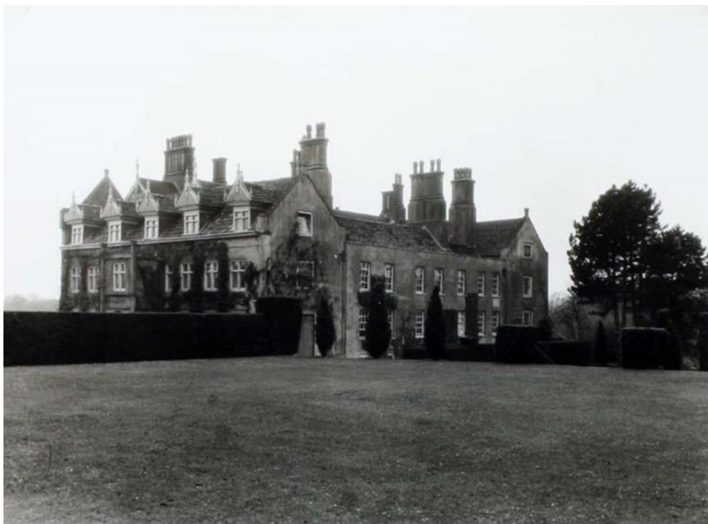
Figure 3.6: East and north elevations of Cuckfield Park, 1884, Historic England The England's Places Collection Card reference no: 5876_003
