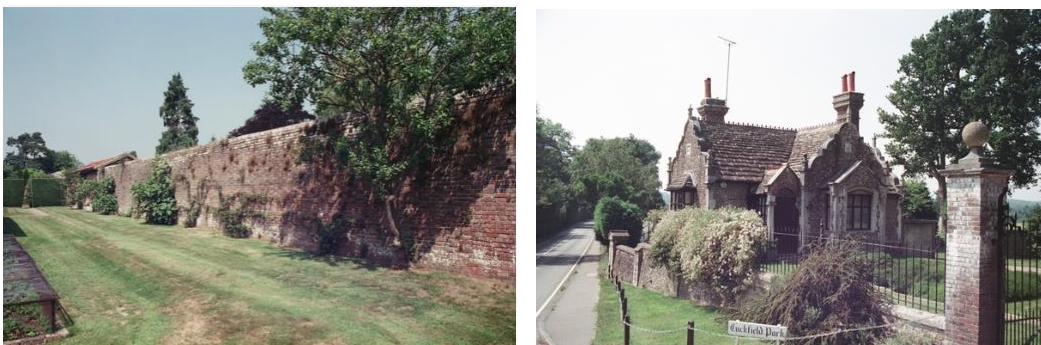
Figure 4.29: Wall to east and south east and Lodge to Brighton Road
