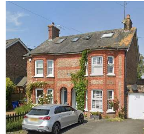
6. Double-height Bay - Buff Multi Brick, Red Quoining
