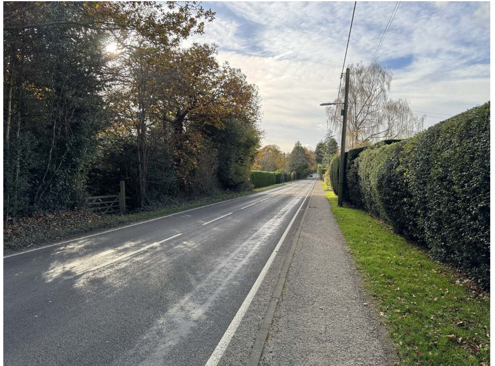
Lewes Road with existing footway on the northern side
