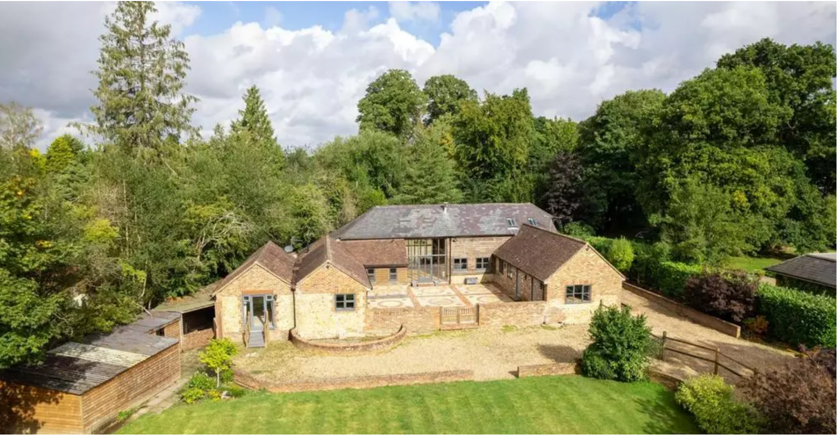
PHOTOGRAPH 5 | North Colwell Barns
