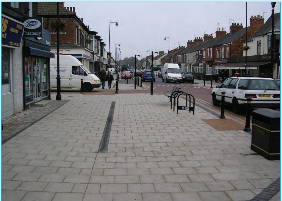
Footways widened significantly by narrowing carriageway
