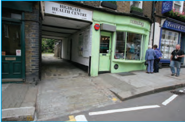
Footway crossover access to commercial premises
