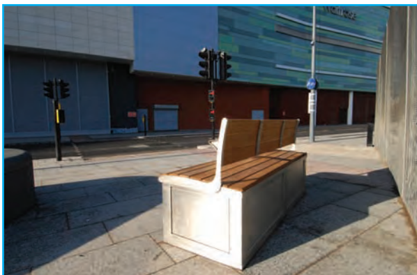
Bench containing traffic signal controller
