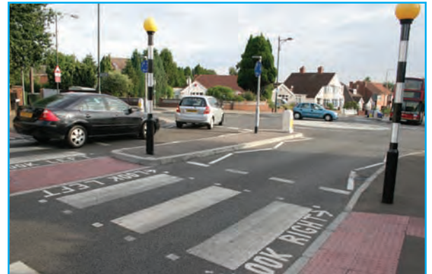
Zebra crossing located close to road junction.
