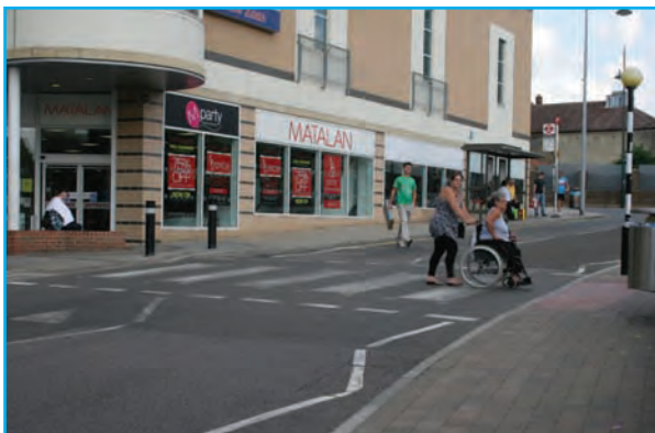
Zebra crossing on raised table.
