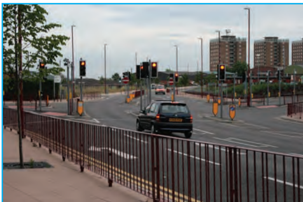
Newly-implemented highway scheme with extensive guardrail
