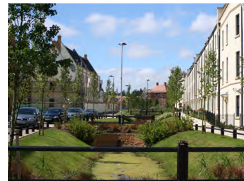
SuDs feature integrated within the streetscene in Upton, Northampton
