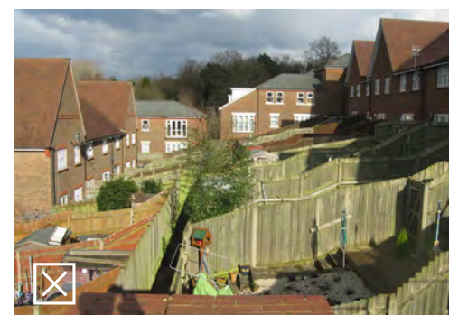
Additional care needs to be taken to accommodate awkward slopes. In this example inadequate consideration has been given to the configuration of the front threshold and the back gardens.
