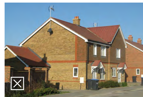
The clay hanging tile is inconsistently applied and appear to peel-away at the side. The roof tile also looks too bright in relation to the facing tile
