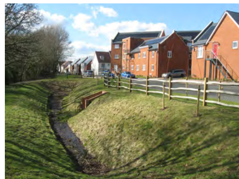
SuDs feature at Maltings Park, Burgess Hill
