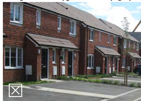
Meter boxes are prominent on building frontages
