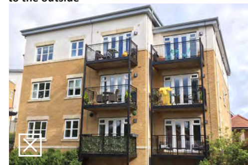
Balconies are inappropriately dominant on the façade and appear to be bolted-on
