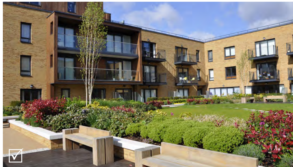
Apartment block benefiting from private communal space
