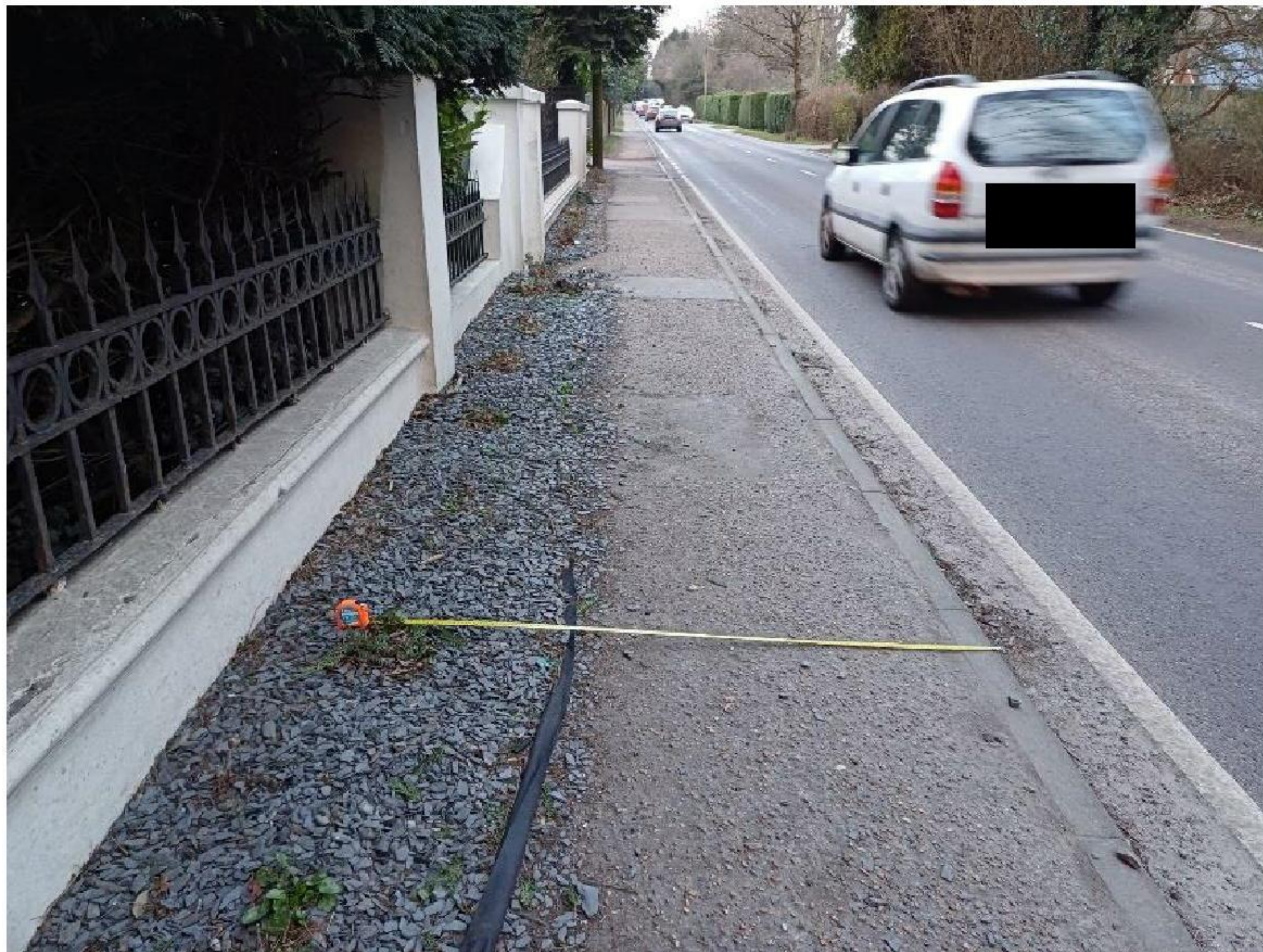
Figure 7 – Lewes Road pavement opposite proposed site entrance (tape measure is set on 1m)
