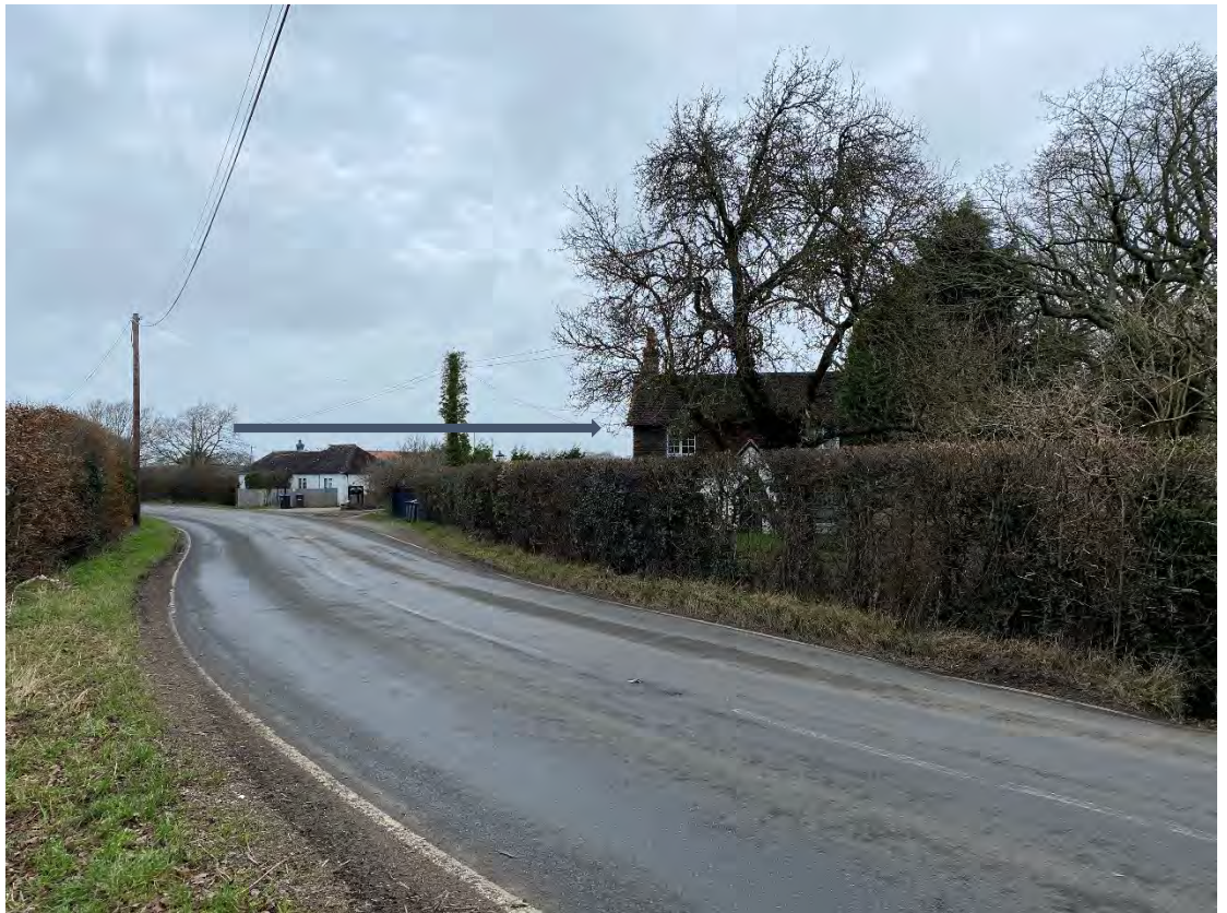
Plate 8 Winter view of the south-east elevation of Westhouse Cottage (Orion 2) from Henfield Road (arrowed).
