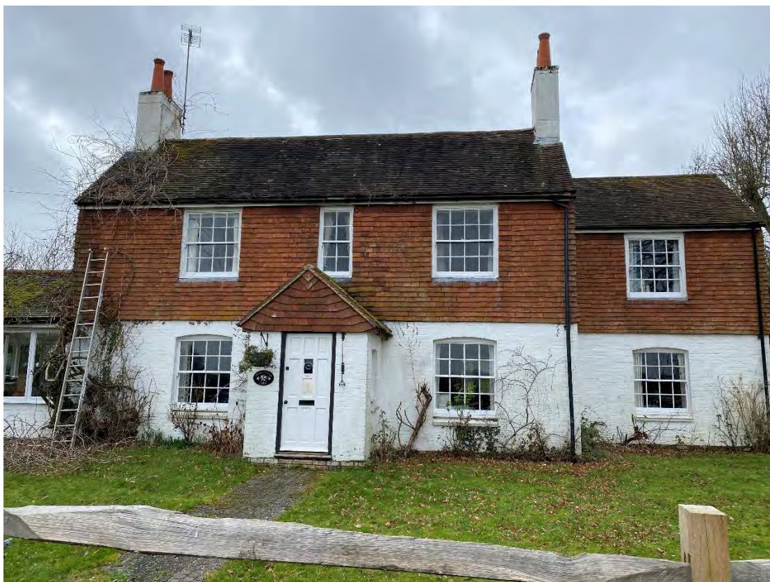
Plate 9 Winter view of the principal (east) elevation of Priestfield Farmhouse.
