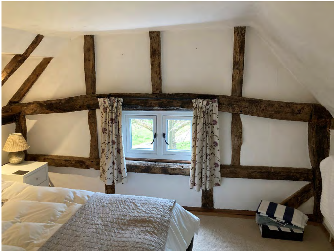
Plate 7 Example of some of the exposed historic timber-framing at first floor level within Gunners (Orion 1).
