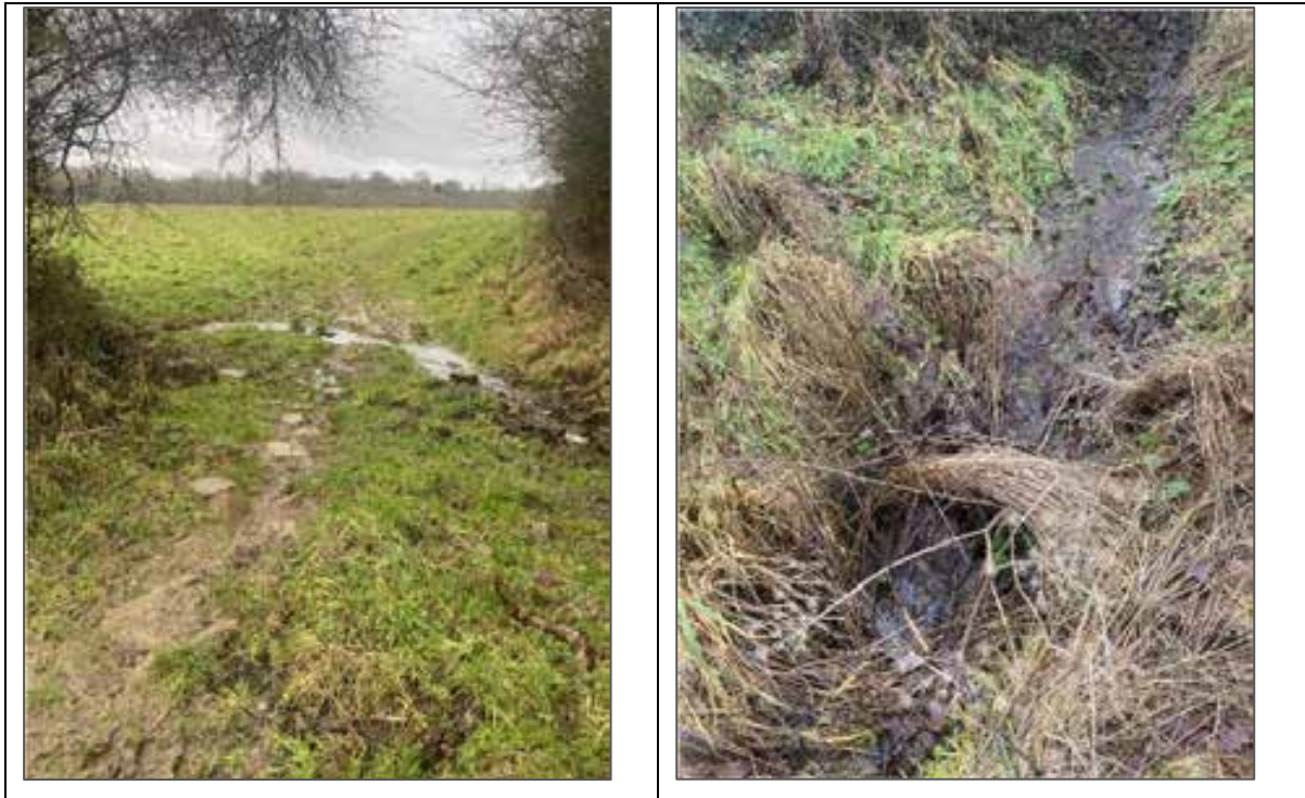
Figure 2-6 (Left) Drain 1 in the north (right) Drain 8
