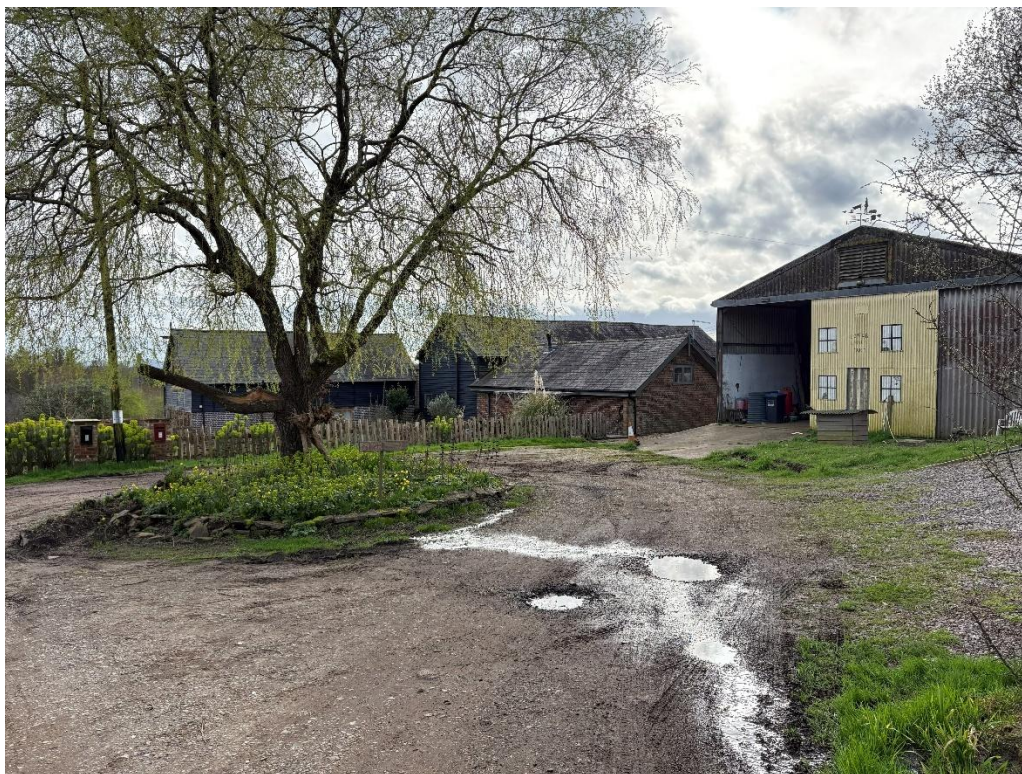
Plate 83 Looking south-west to the farm buildings of Laines Farm
