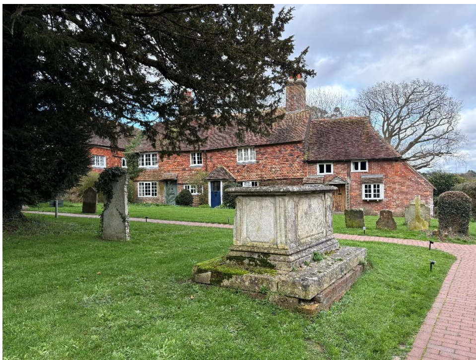
Plate 63 Cottages to the east of the churchyard
