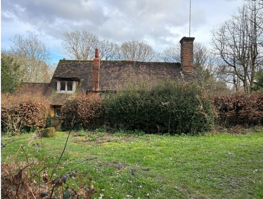
Plate 34 Looking south-east to Mackrells Cottage
