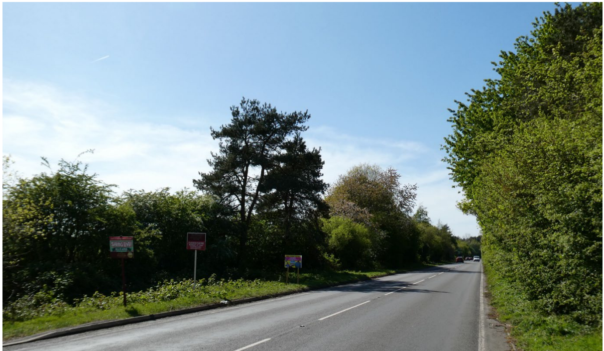
Figure 9 View along the A272 looking west towards the Cuckfield B2036 roundabout showing the location of the northern vehicular access with a signalled crossing, the Appeal Site to the left of the view and the extent of the proposed cycle route visible along the A272.
