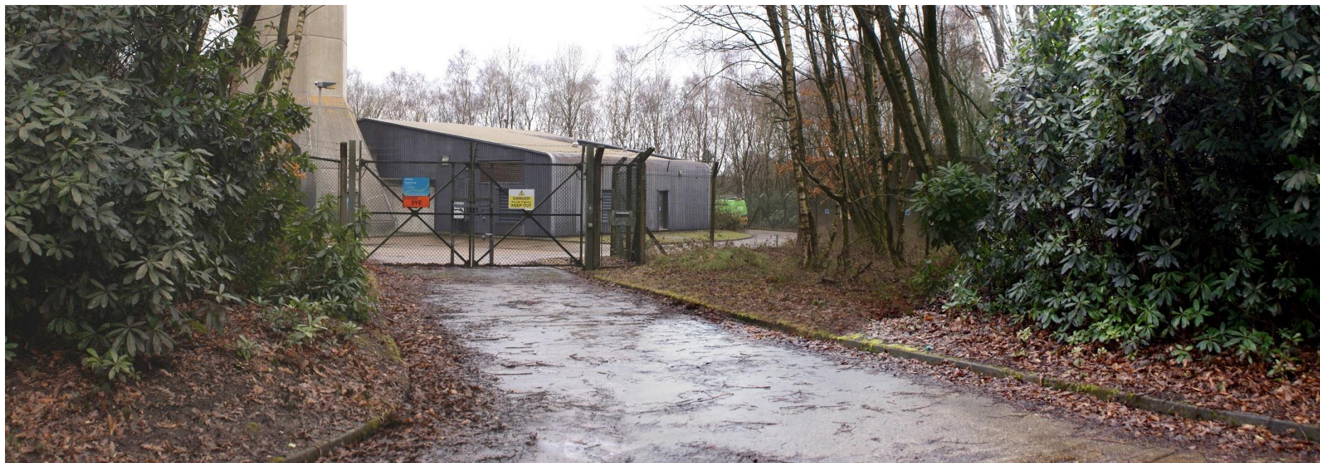
Viewpoint (panorama) 5: Near view east from public bridleway 1546 which follows the route of the access road north from Horsham Road to Cottessmore School. The view is dominated by the base of the NATS radar tower and associated building, signage, gates, fencing and tarmac access. Views to the rear are largely screened by trees. There are no views of the Site.
