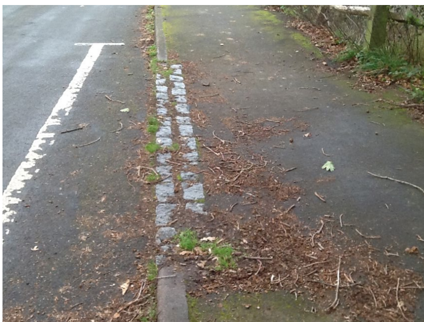
Figure 1 - dropped kerb at entrance to SA29
