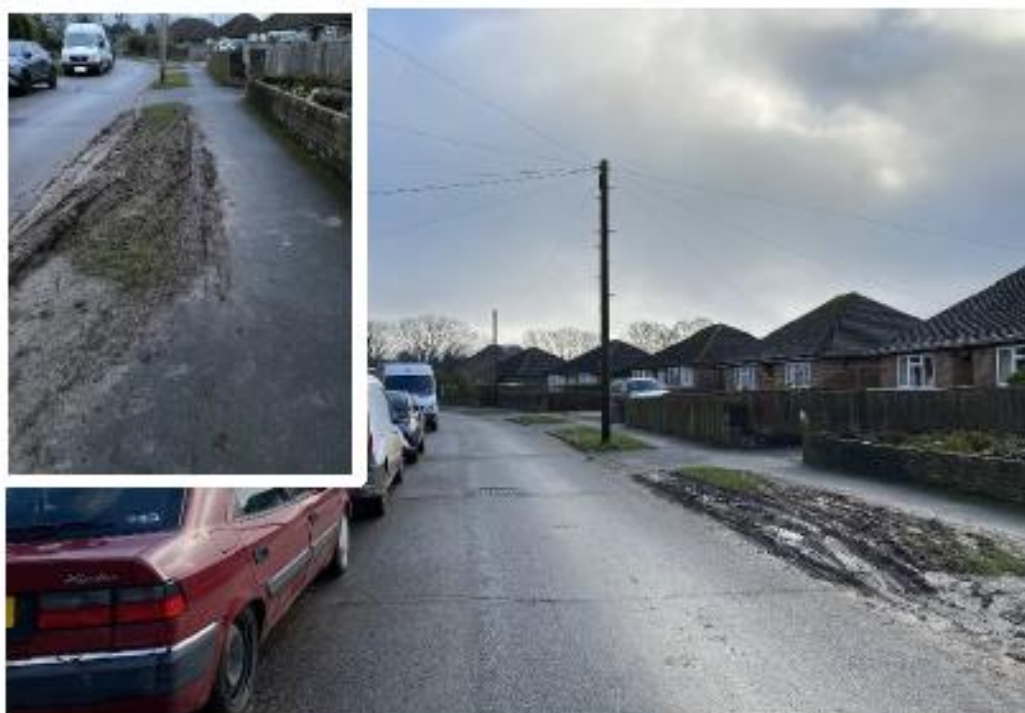
Figure 3: Evidence of frequent driving on grass verge and pavement along Hamsland as a result of head-to-head conflicts (View looking east along Hamsland c.75m east of Lewes Road junction. Friday 5 th February @ 9:22; Inset Monday 22 nd February @ 17:34)
