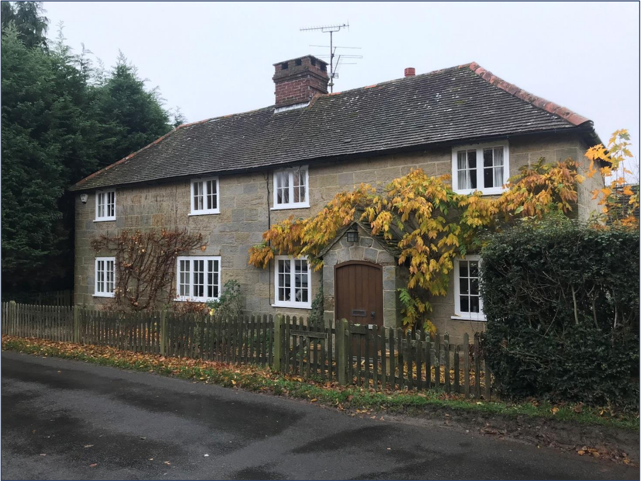
Plate 4: Knowles Farmhouse on the south side of Street Lane.
