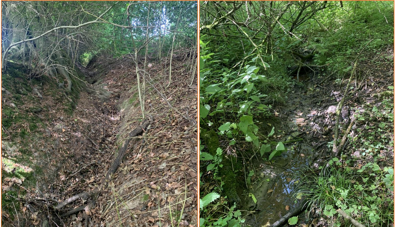
Figure 6: Photos of the Downstream Section of the Centre North Drainage Ditch (Source: Unda Consulting Ltd)
