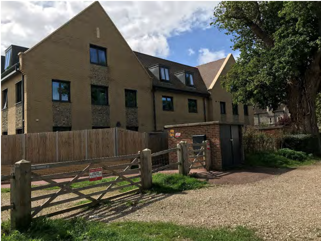
Plate 9 Modern development in immediate setting of the listed buildings at Hurstpierpoint College
