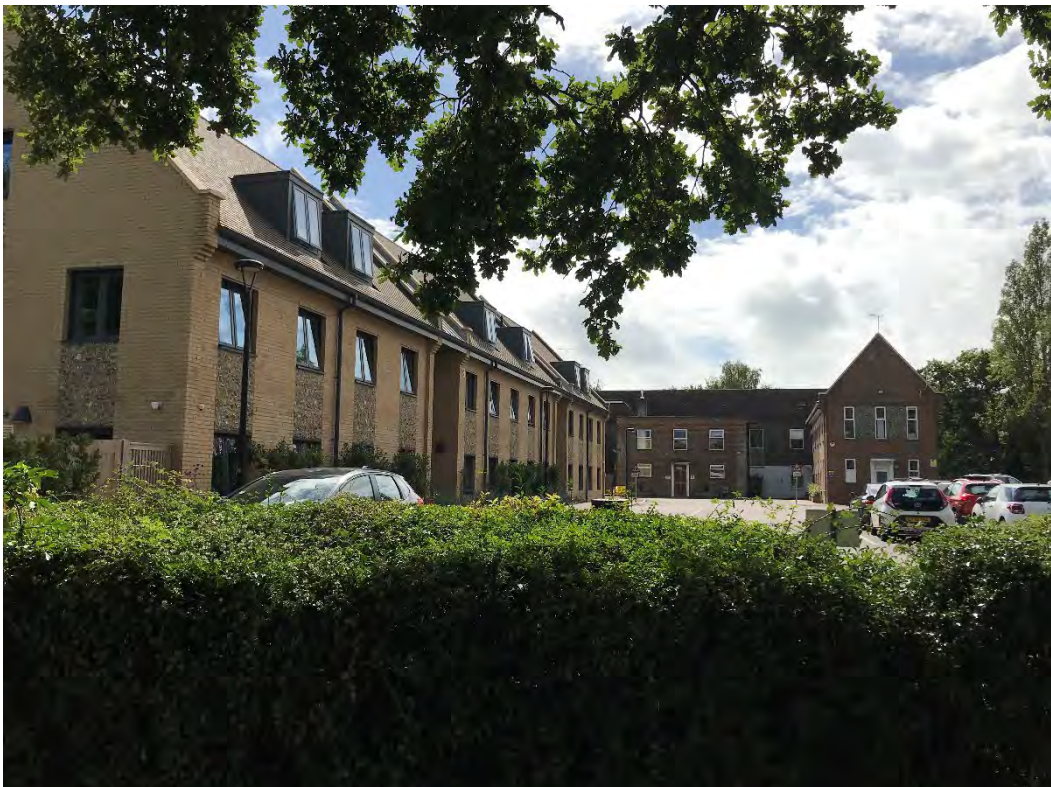
Plate 10 Modern development in immediate setting of the listed buildings at Hurstpierpoint College
