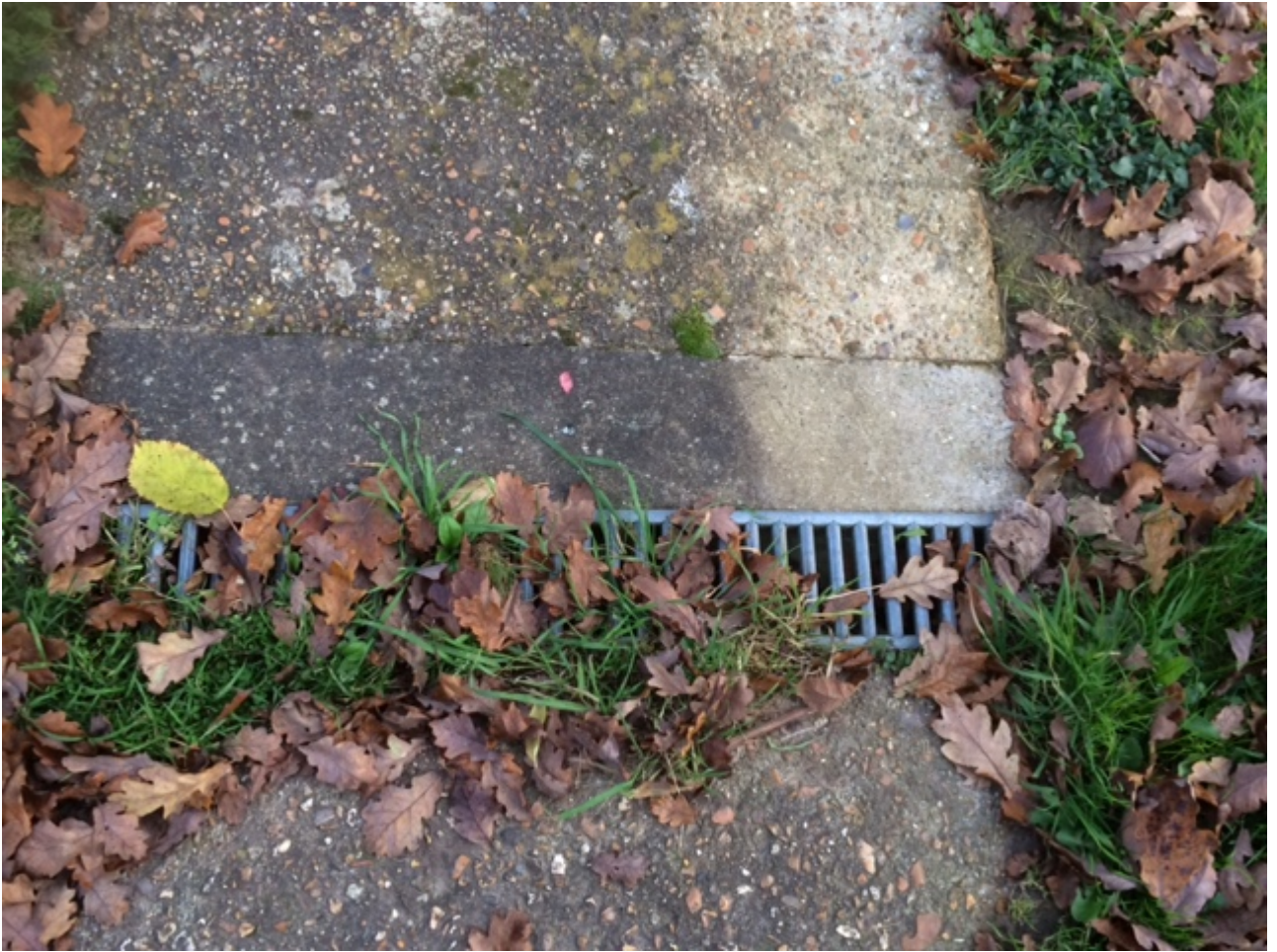
Drainage installed due to run off water from the site.
