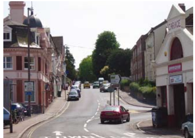
ABOVE: Boltro Road, Haywards Heath
