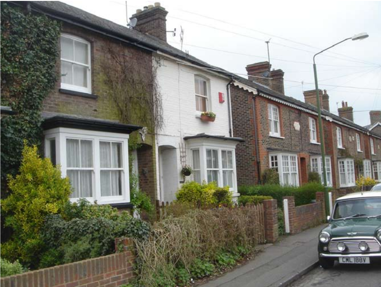
ABOVE: Hayward Heath has some attractive Victorian buildings
