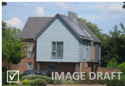
Contemporary chimney designed to provide ventilation but also articulate the roofline
