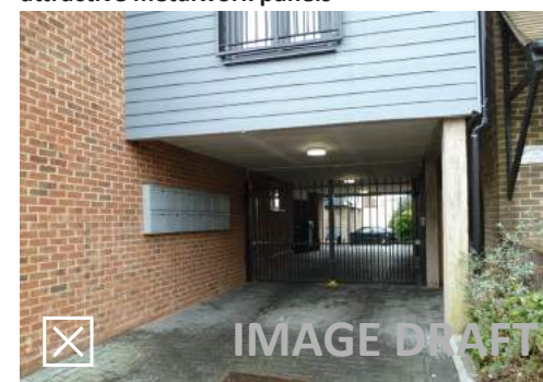
Access to undercroft car parking is discretely located on the street however the setting back of the gate presents a security risk
