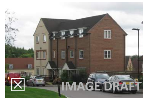
Little thought has been given to the positioning of rain water pipes, which is especially an issue when the eaves line is broken
