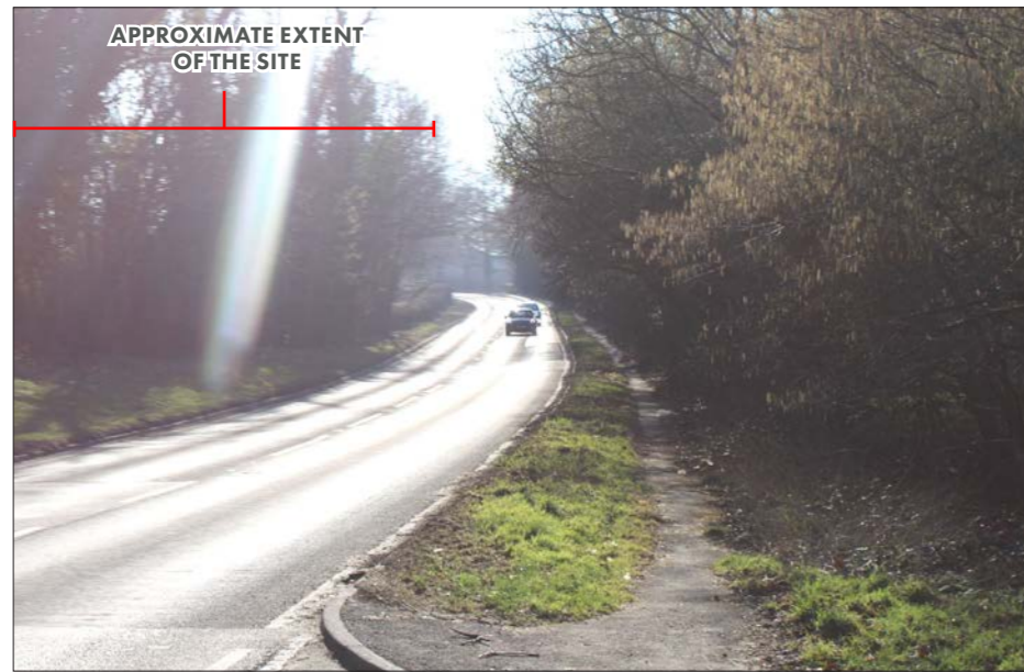
PHOTOGRAPH - VIEWPOINT 9 CONTINUED
