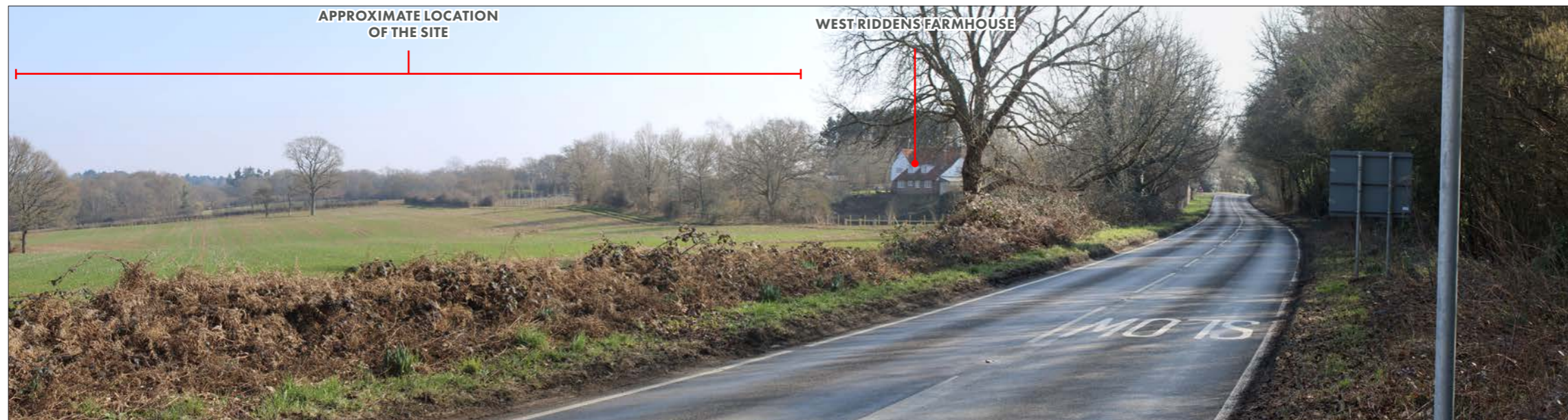
PHOTOGRAPH - VIEWPOINT 40 CONTINUED
