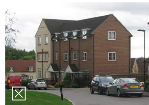
Little thought has been given to the positioning of rain water pipes, which is especially an issue when the eaves line is broken
