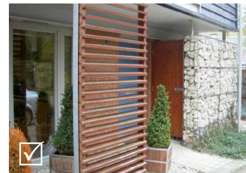
Refuse areas should be considered as part of the design of the buildings. If refuse areas are located to the front of the building they should be designed as an integral part of the elevation
