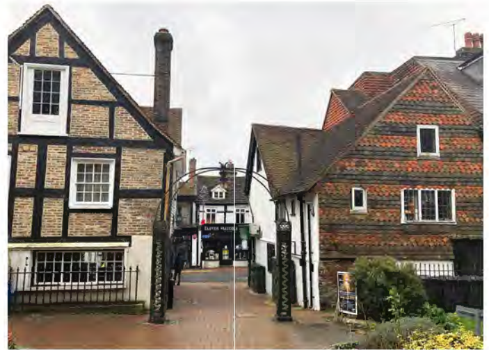
View South from Church of St Swithun
