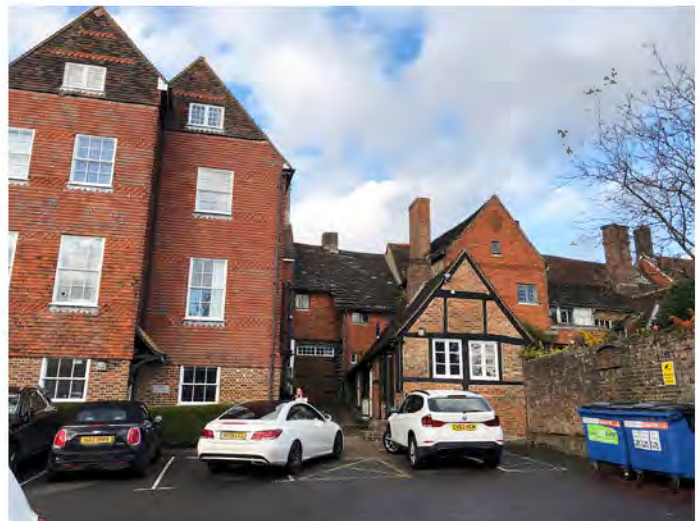
Rear of 58-64 High Street
