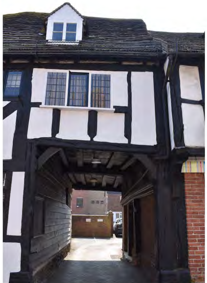
Carriageway between 46 and 48 High Street
