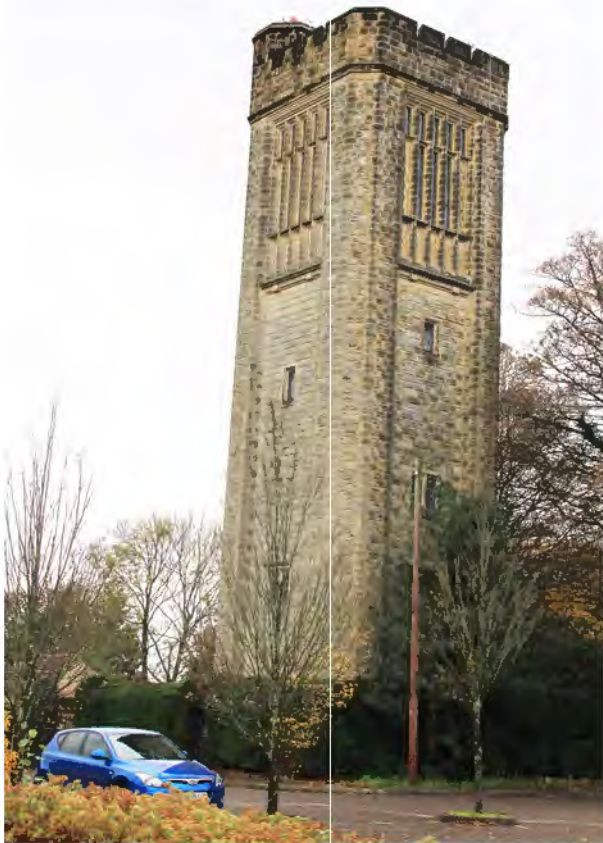
Sackville Water Tower, Church Lane
