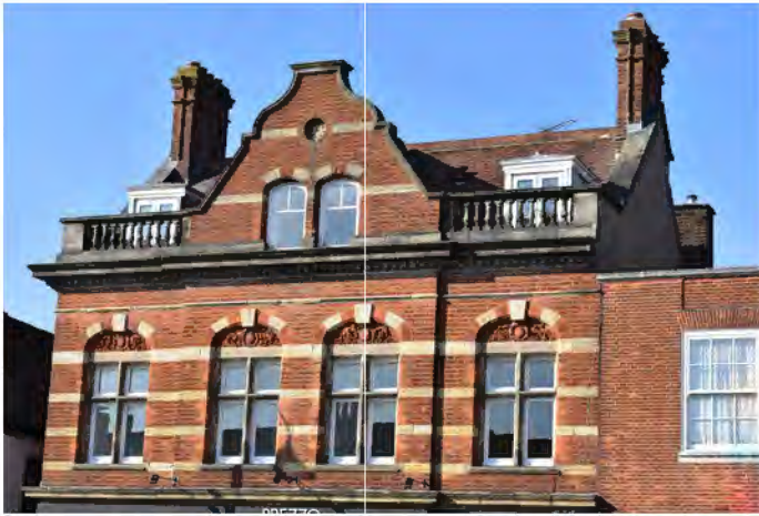
Polychromatic brickwork on 13 High Street
