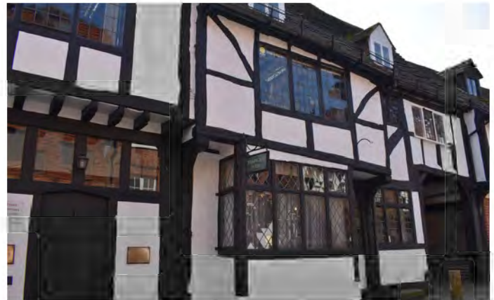
Wilmington House, 48 and 50 High Street
