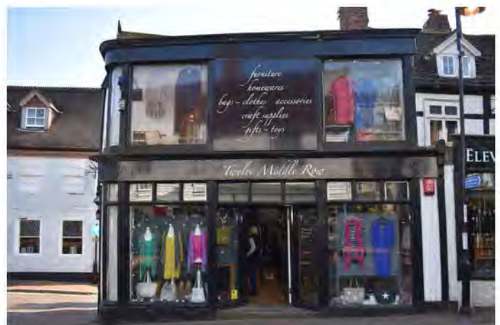
12 Middle Row: Positive shopfront
