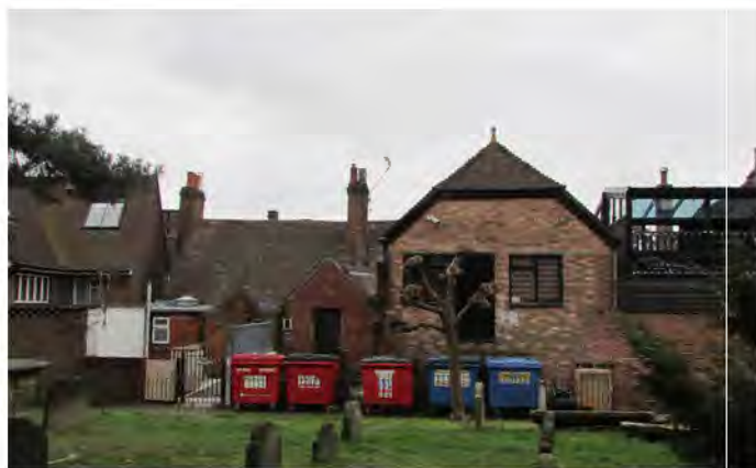
View south of Church at unsightly waste to rear of High Street
