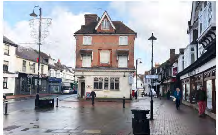
View of the Former Midland Bank, from West of High Street
