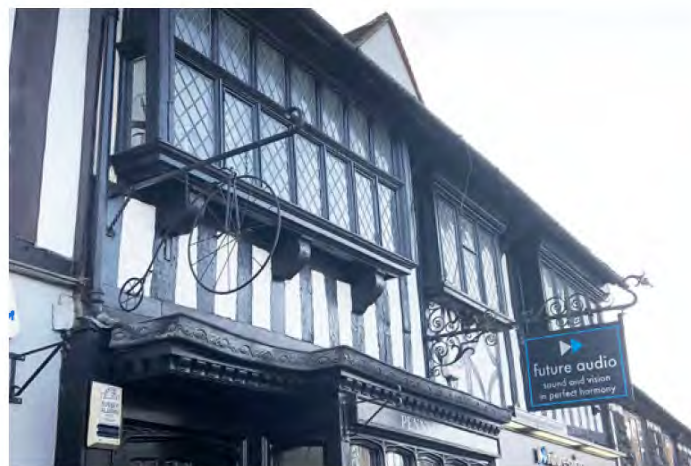
Oriel windows, 30 High Street
