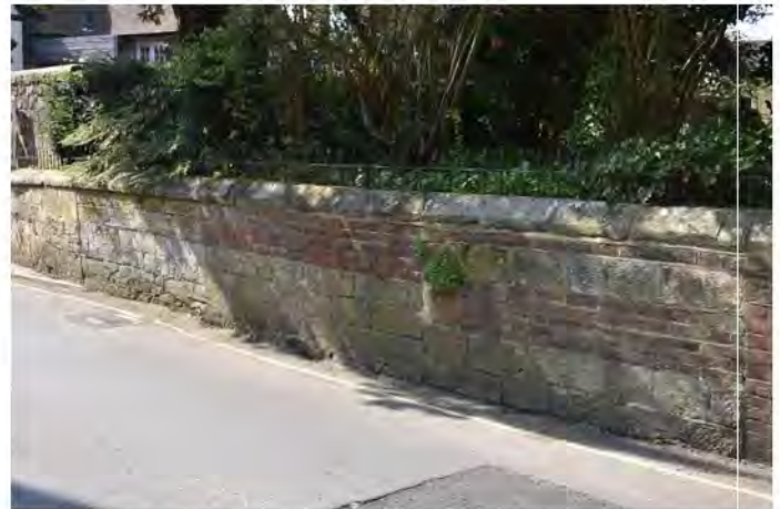
Wall at Eastern boundary of Church of St Swithun
