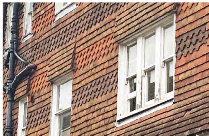
Tile hanging - The Old Midland Bank, 1 Middle Row
