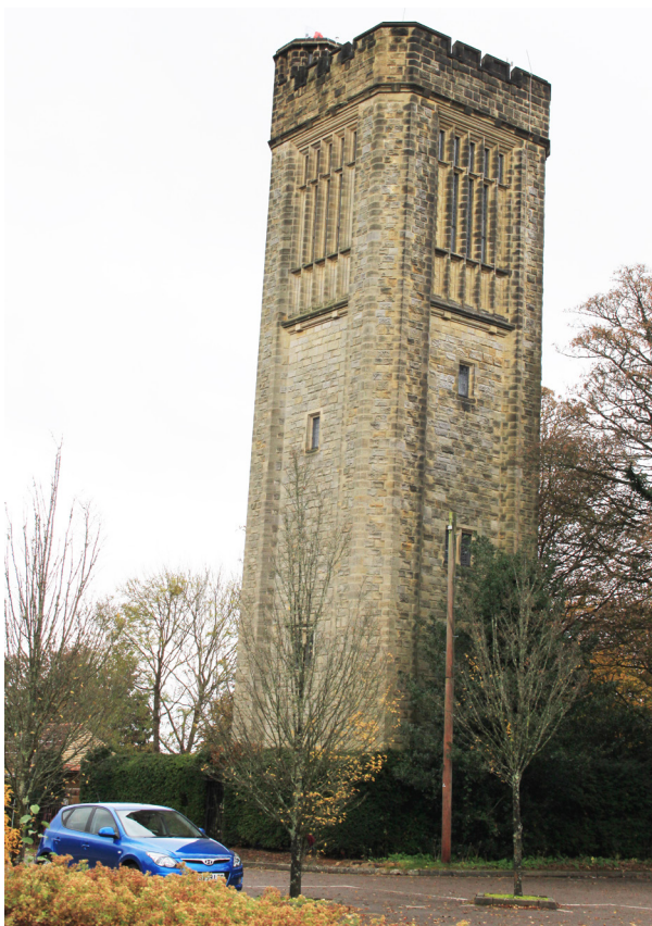
Sackville Water Tower, Church Lane
