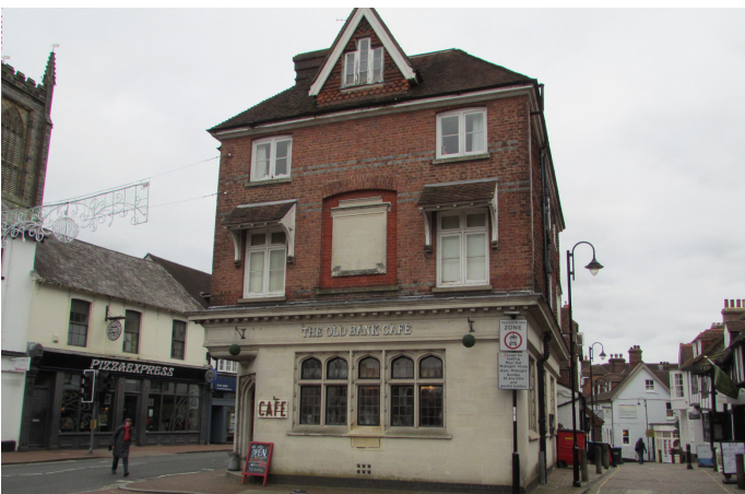
Former Midland Bank, 1 Middle Row
