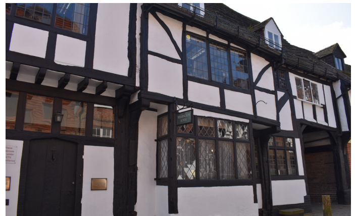
Wilmington House, 48 and 50 High Street
