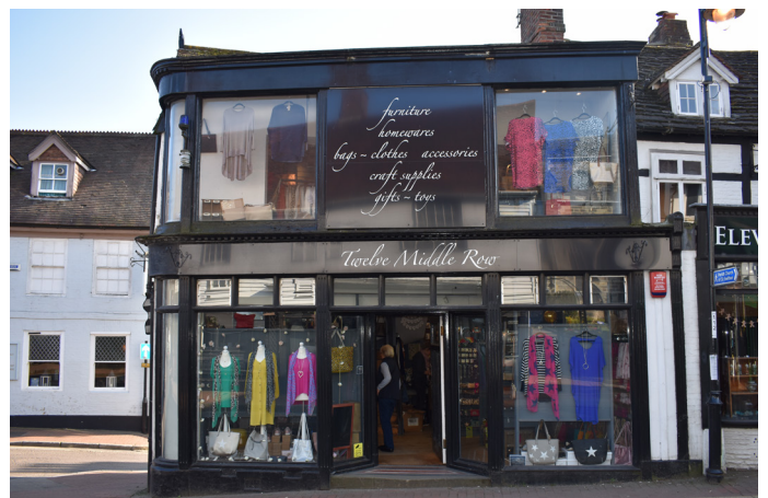
12 Middle Row: Positive shopfront
