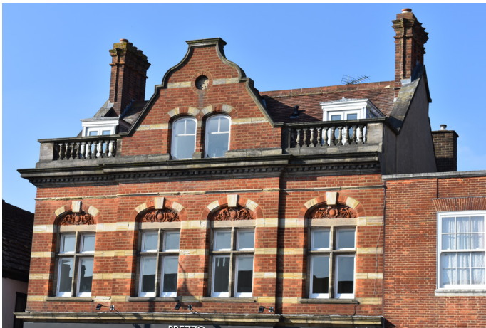
Polychromatic brickwork on 13 High Street
