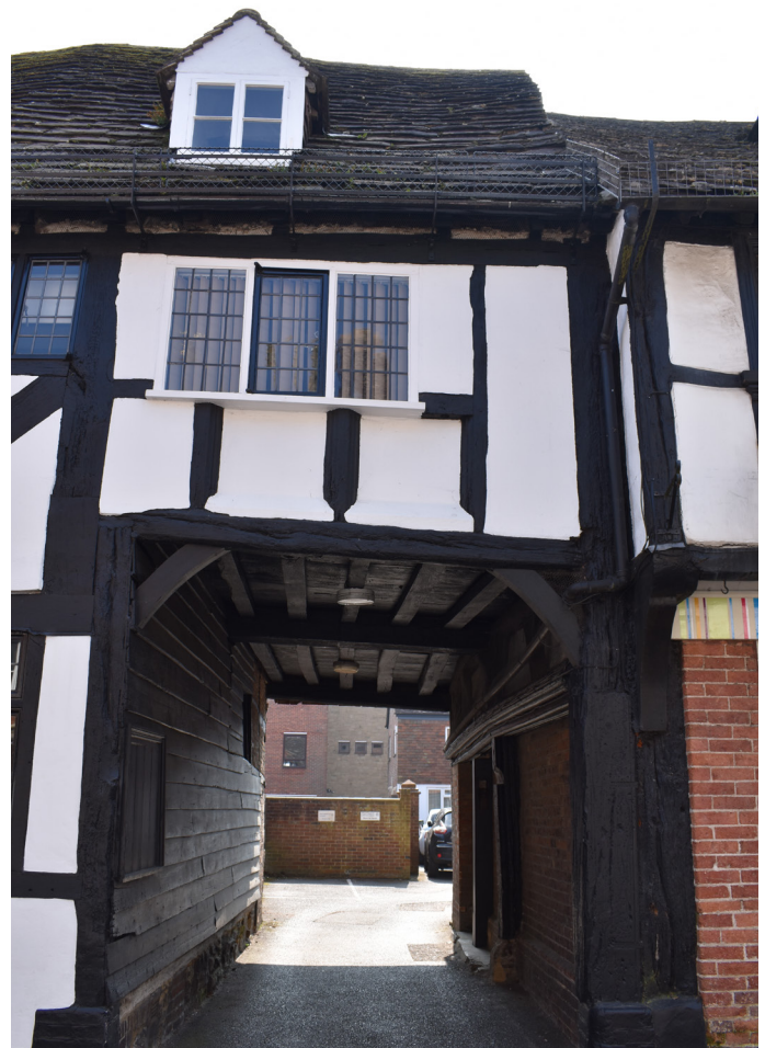
Carriageway between 46 and 48 High Street
