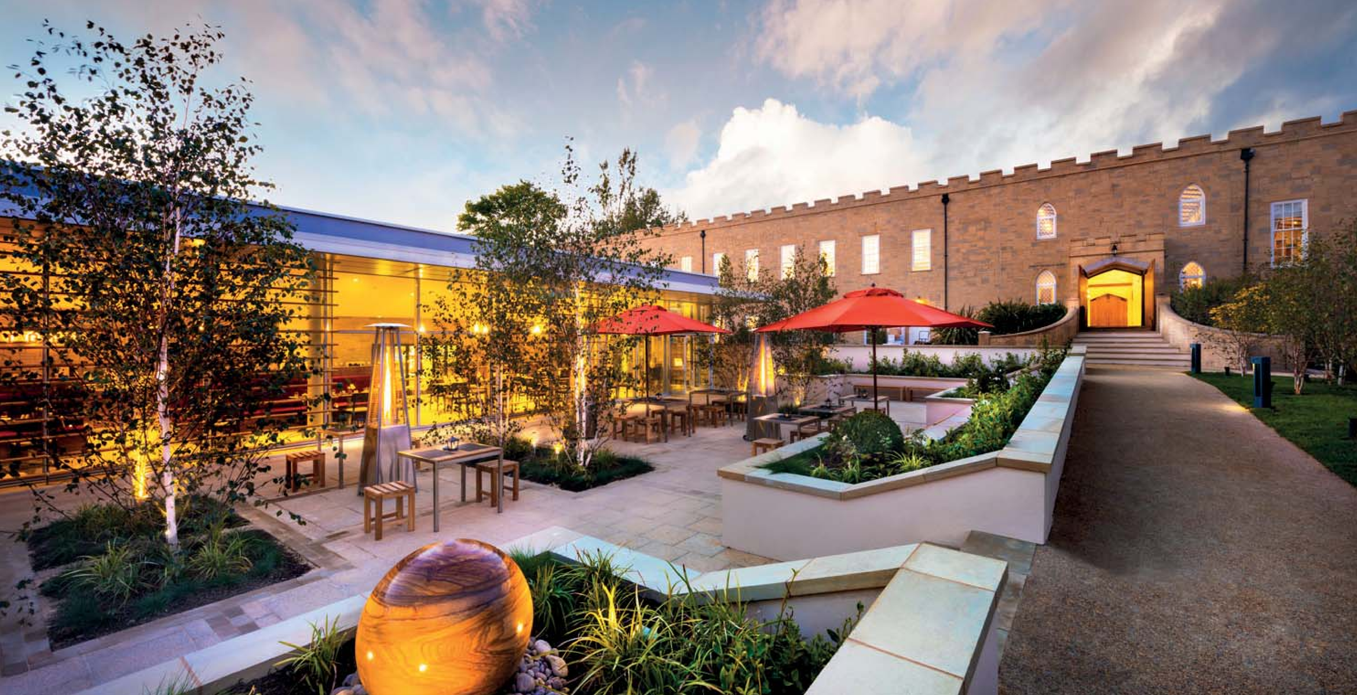
Photo provided by Client
