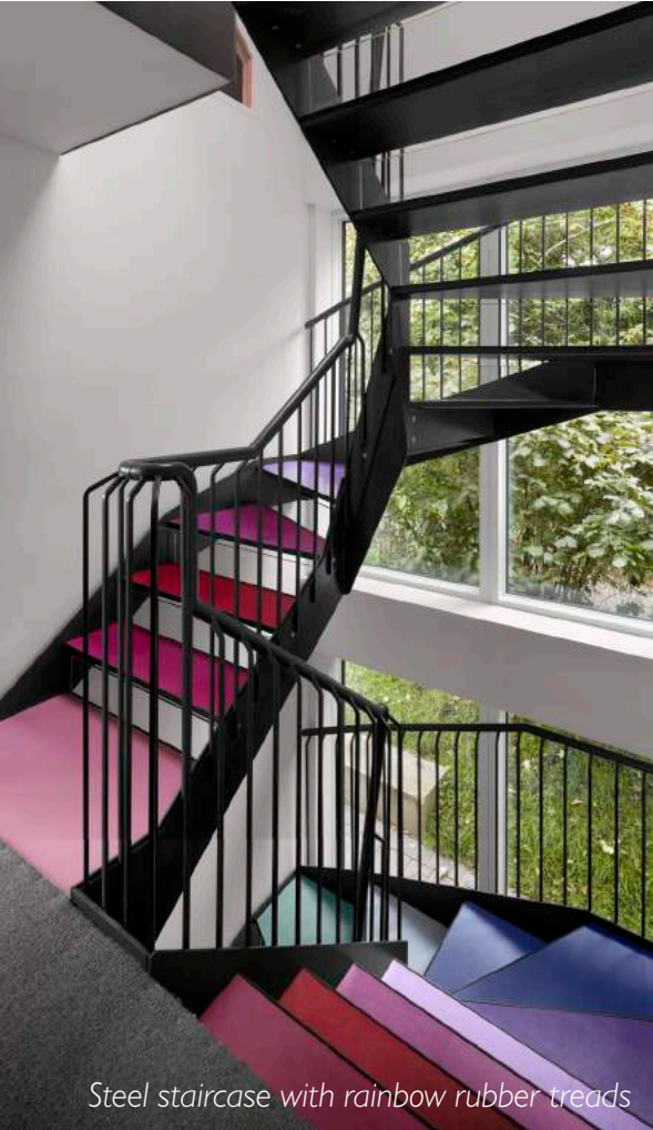
Steel staircase with rainbow rubber tracks
