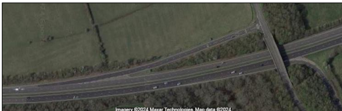
Figure 23. Aerial view of existing A23 B2117 – Southbound on-slip
