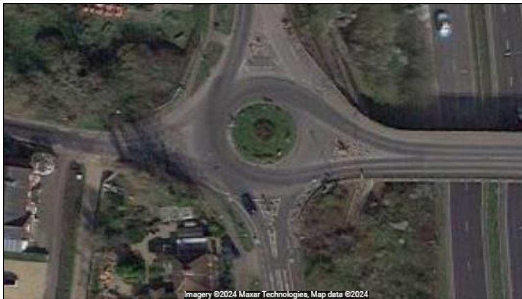
Figure 15. Aerial view of existing Hickstead Interchange West junction layout
