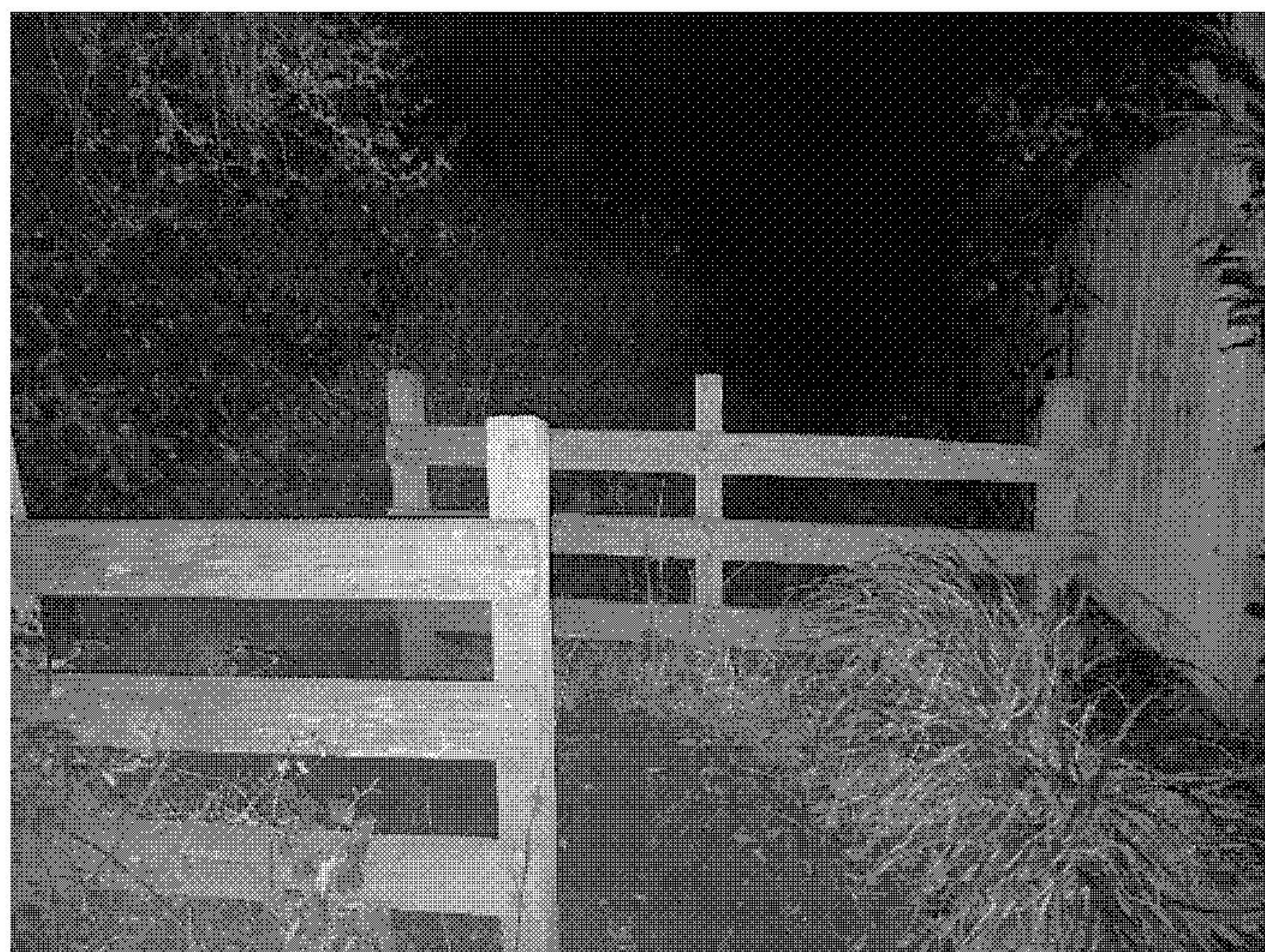
Figure 5: Uneven sections of 29CU footpath
