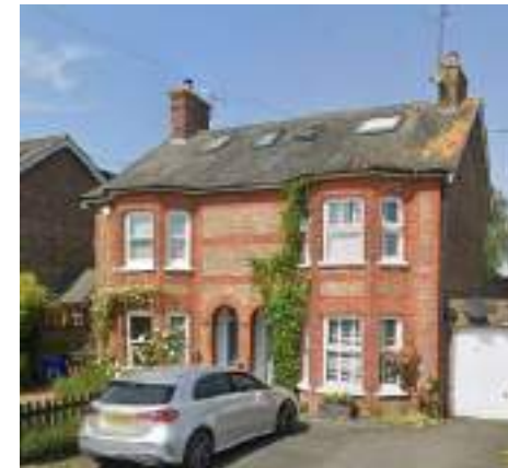
6. Double-height Bay - Buff Multi Brick, Red Quoining
