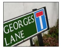
Nameplates should be constructed using a die-pressed plate in galvanized frame painted black with 90mm or 50mm white 'Kindersley' uppercase lettering on a green background with white border. The height of the plate should be 150mm for single line text.
