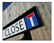
Nameplates should be constructed using a die-pressed plate in galvanized frame painted black with 90mm or 50mm 'Kindersley' uppercase lettering on a white background with black border. The height of the plate should be 150mm for single line text.
