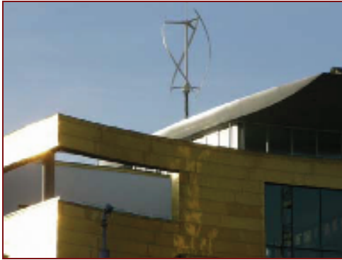
Vertical axis rooftop turbine (6kW)
