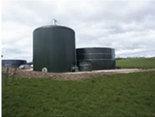
Farm scale anaerobic digestion plant
