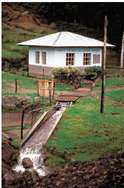
Small scale hydro plant
