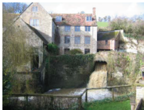
Small scale hydro plant at an old mill site
