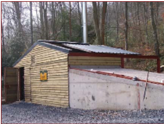
Small scale wood fired boiler plant
