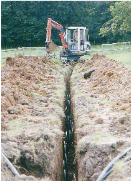
Trenched ground loop for ground source heat pump
