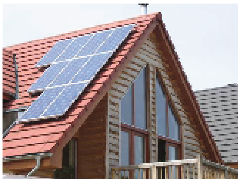
Retrofit PV panels
