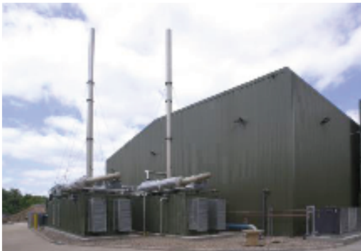
Wanlip waste to energy plant (1.4 MWe)
