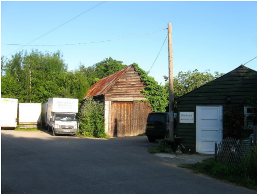
Glebe Farm Industrial units
