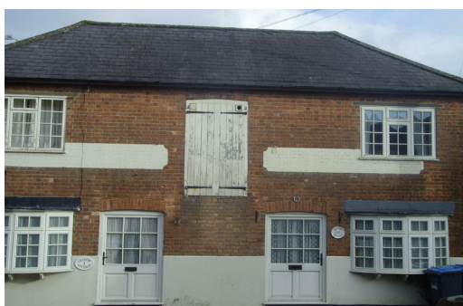
Granary Cottages, Village Centre
