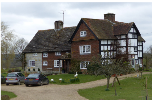
Spicers, a Balcombe Estate owned rental property
