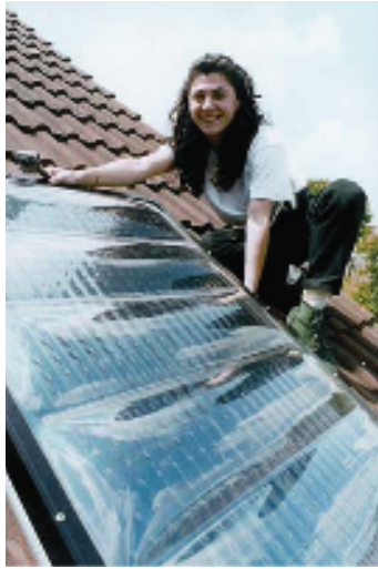
Solar thermal panel
