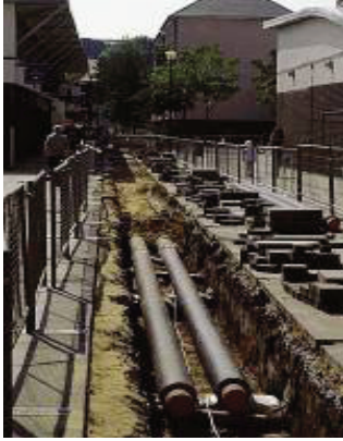
Installation of district heating pipes under road
