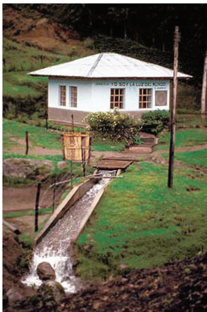
Small scale hydro plant
