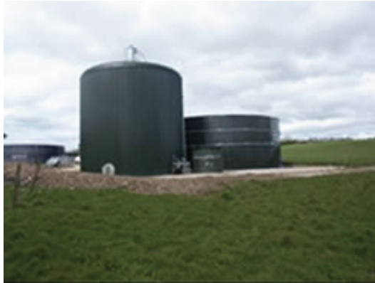
Farm scale anaerobic digestion plant
