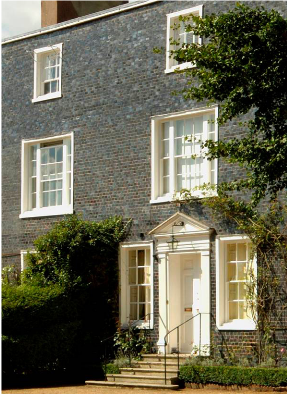
Fig. 18. Mathematical tiles used for the early 19 th -century re-fronting of 17 th -century 141-3 High Street.
