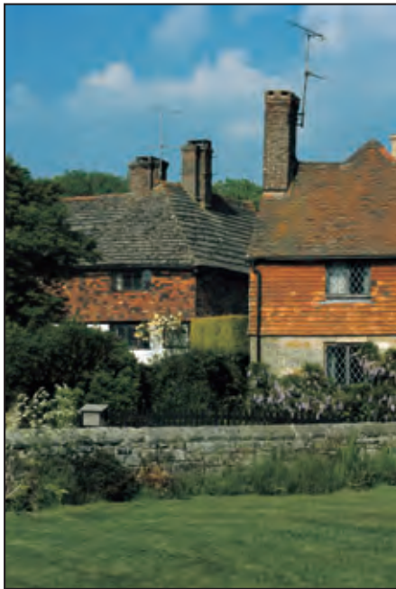
Traditional buildings reflect the use of local materials, such as redbrick and tiles,
