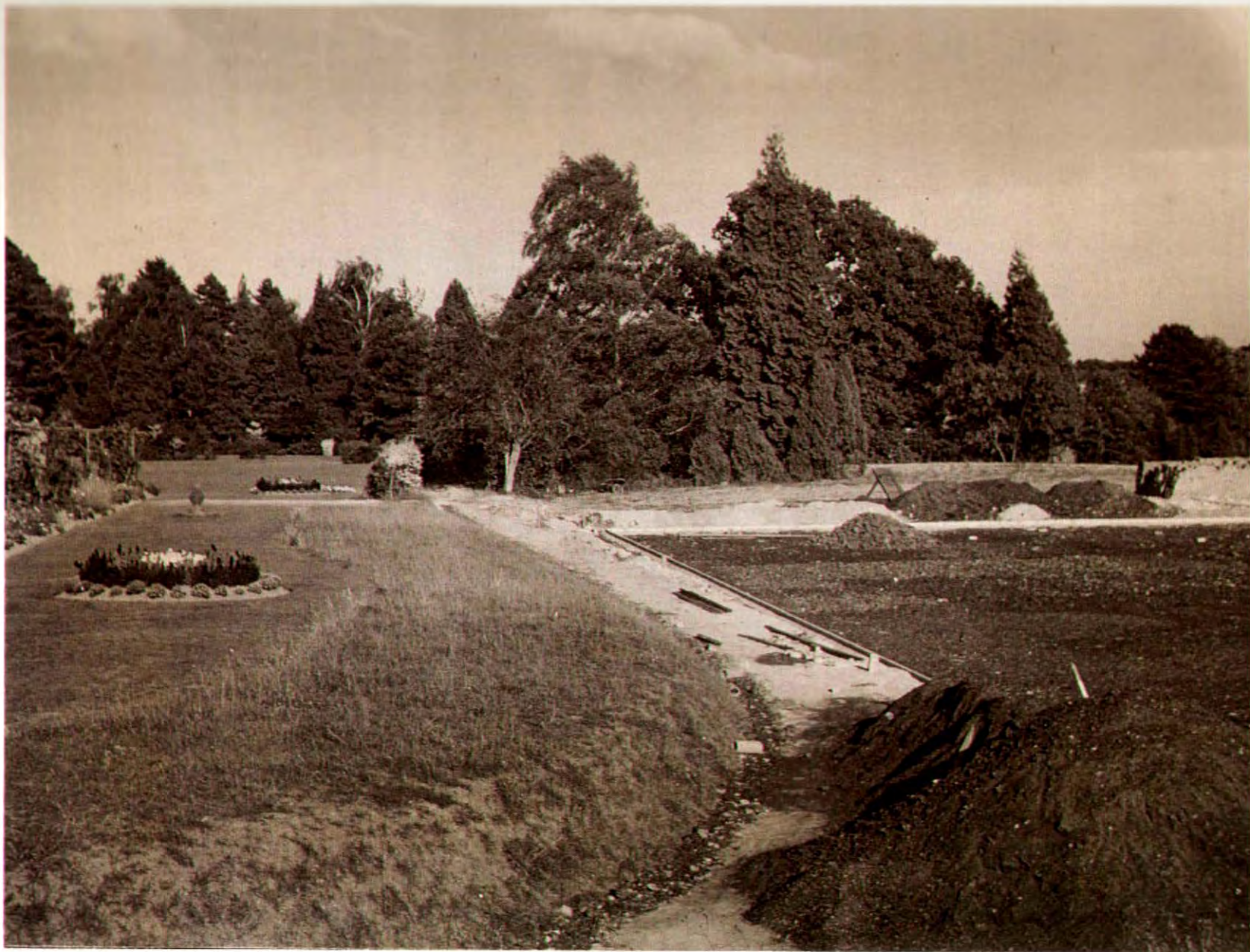
Figure 10 - View looking east. April 1952.
